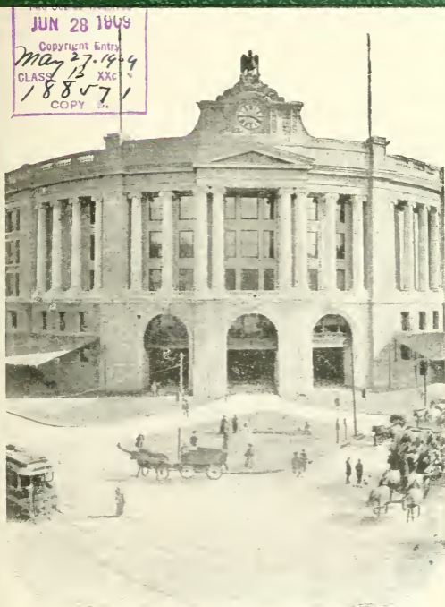
South Terminal Station
